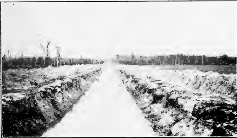
FIG. 1.—SLOPE COURSE OF MUD CREEK DREDGED CHANNEL, NEAR TUPELO, MISS., 1913. (SEE TABLE NO. 1.)
